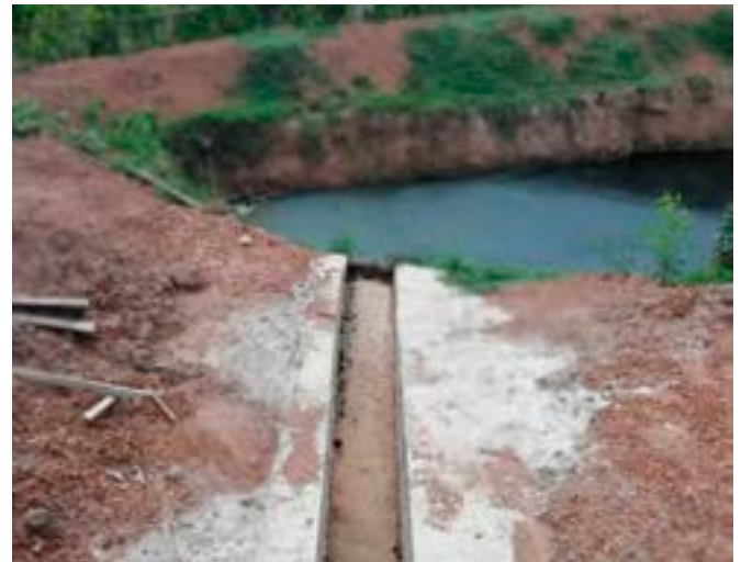
Dao's new pig shed was designed with help from the District Agriculture and Forestry Office. The sloping concrete floor makes it easier to keep the pens clean, and slurry is channelled into a pond where it is stored until the dry season to be spread on nearby rice fields.
